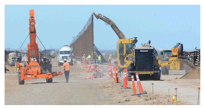
A construction worker (left) helps move a section of reinforcing grid into place while a trenching machine (right) digs a new footing and other construction workers assemble a 30-foot-high bollard style wall at a construction site south of Yuma, Ariz., near the border between the United States and Mexico.(Randy Hoeft / AP)
